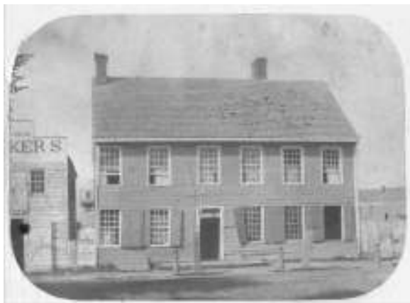
This photograph of the building was taken just before it was demolished.
